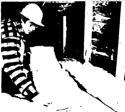
Manufacture and installation of insulation are booming.
